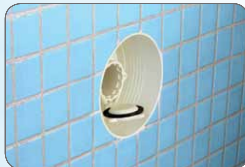
Remove Dress Ring Cover, open spring loaded port.
